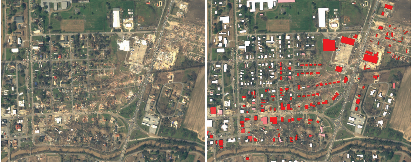
Figure 1. (Left) Post disaster Planet SkySat imagery over Rolling Fork, Mississippi from March 25th; (Right) Building level model damage estimates (color gradient indicates damage from no damage colored in white to destroyed in red).
