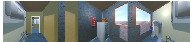
Figure 18. Panorama view of the service shaft room.
