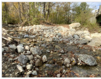
Upstream of abutment 2
