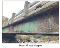
Beam #5 near Midspan
