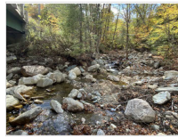
Upstream of abutment 1
