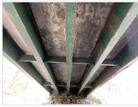
Deck & superstructure abutment 2
