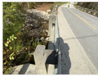
Upstream rail from abutment 1
