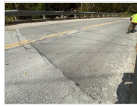
Deck & upstream rail from abutment 1
