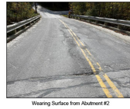
Wearing Surface on Abutment #2
