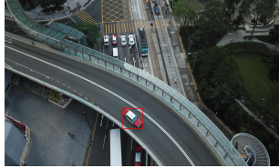
The red taxi travels on the elevated roadway.
