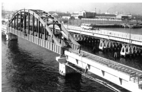
A train crossing a bridge over a river
