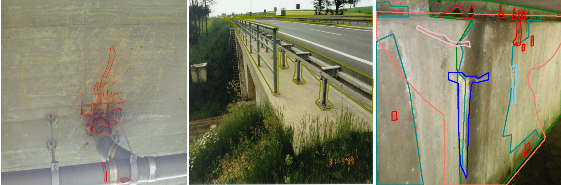
(a) No clear border of the defect ( Rust ), the class ( Protective Equipment ) is stretched from fore- to background. Many overlapping classes with partially low contrast like the border and hatching of the Hollowarea (pale red), and the Efflorescence (dark blue) next to the bright, dry and healthy concrete surface.
