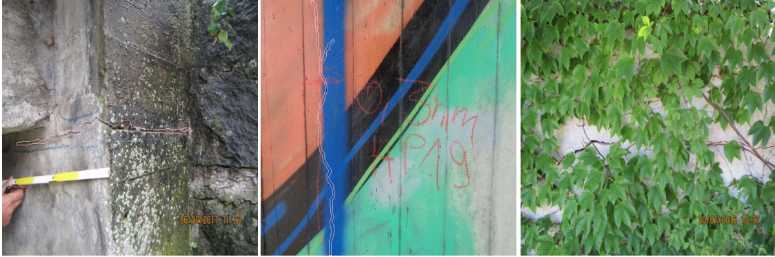
(a) Challenging samples showing a Crack : in combination with strong Weathering , in combination with Graffiti and partially overlapped by vegetation ( Weathering ).
