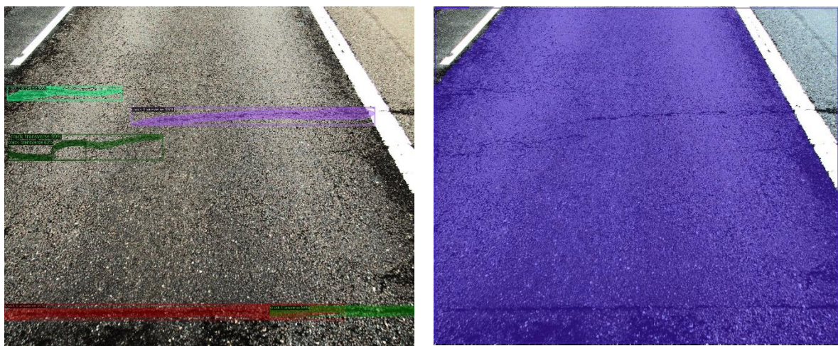
Detection using Mask R-CNN (trained with 1614 positive images with 2335 instances)
