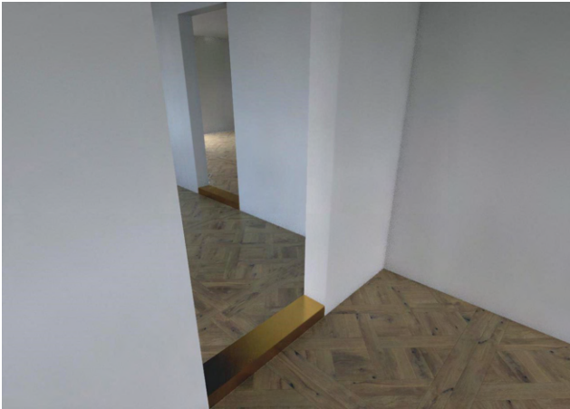
Figure 9. The low-height gold-colored thresholds act as obstacles that may pose a danger to the users.
