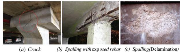
Figure 1. This paper only concerns the crack(a), spalling with exposed rebar(b), and pure spalling(c) three kinds of concrete flaws. The condition states of these flaws consist of CS1 (good), CS2 (fair), CS3 (poor), and CS4 (severe) four degrees.
