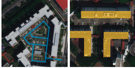
Figure 1: Example of correlations between carparks and other geographic objects, i.e. , roads (left) and buildings (right). Original Images © 2018 Maxar Technologies Inc.
